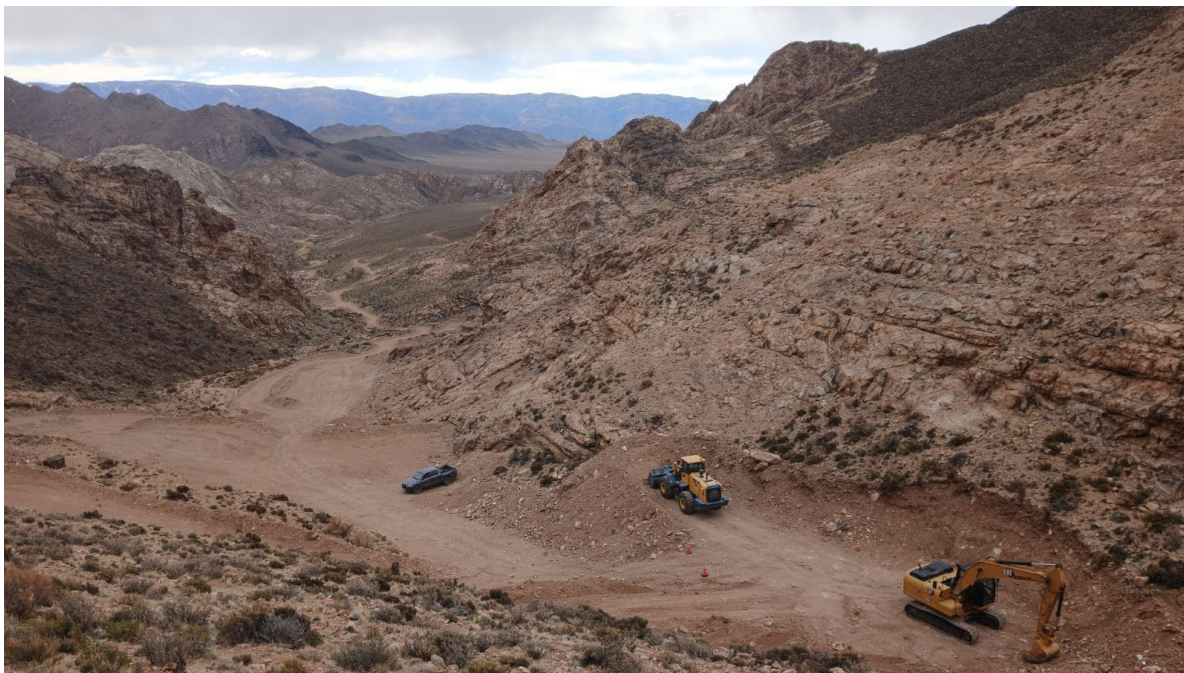
Figure 3: Earthworks underway ahead of Phase 2 drilling; access being prepared to southwest of 26-LODH-023, following the geologic structure up the gully
