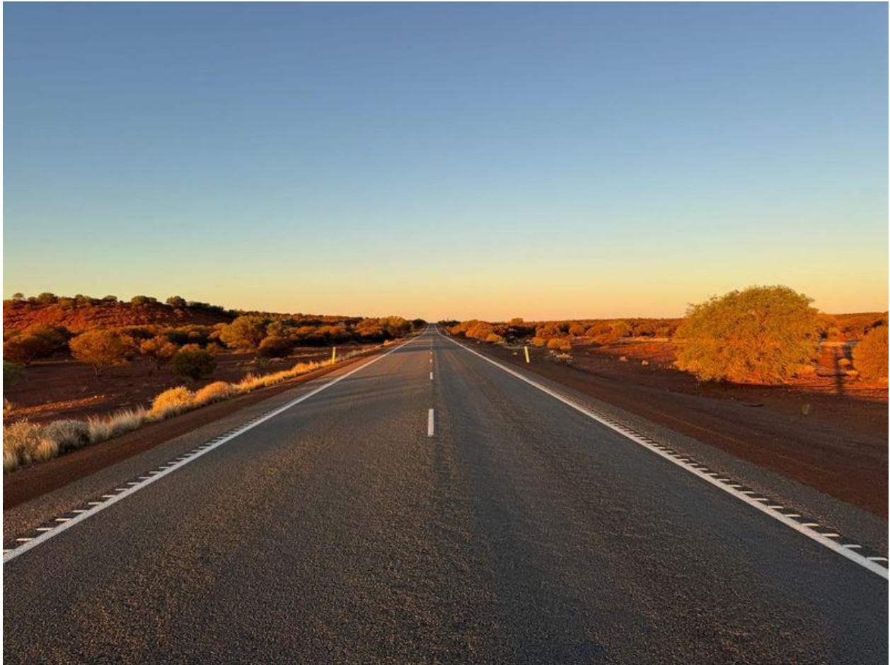
Figure 9 - Great Northern Highway looking North
