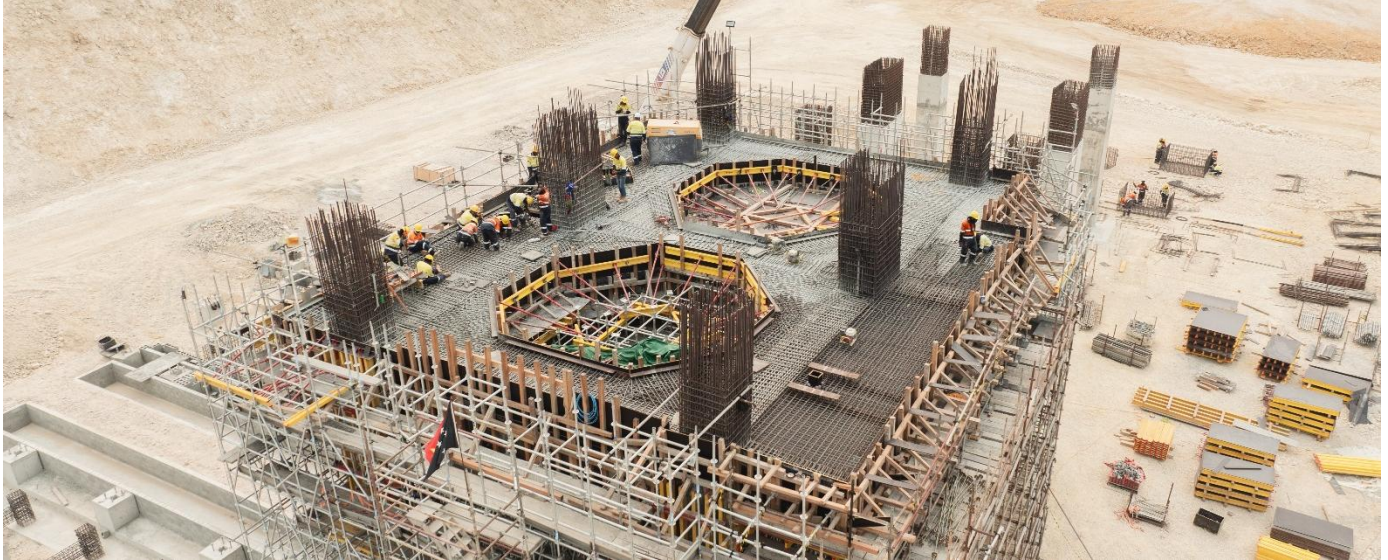
Image: Reinforcement being placed on the Kiln 1 raised support deck, September 2026
