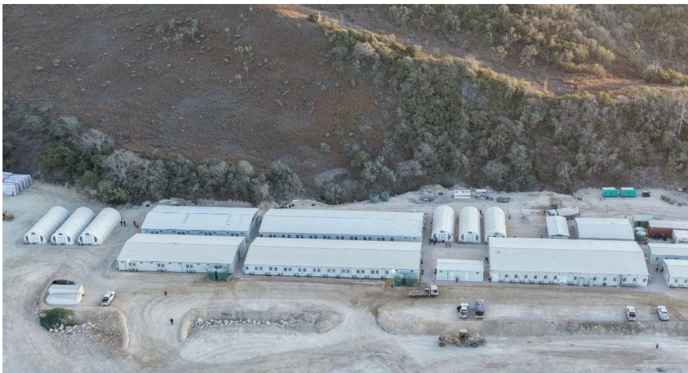
Image: Expanded construction camp accommodation
