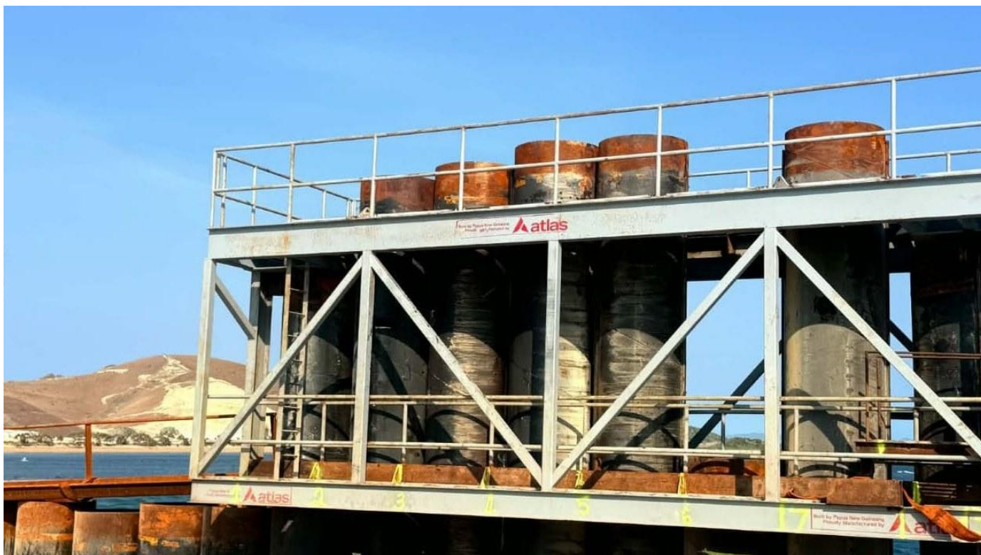
Image: Multi-pile frame in position for Phase 3 wharf piling
