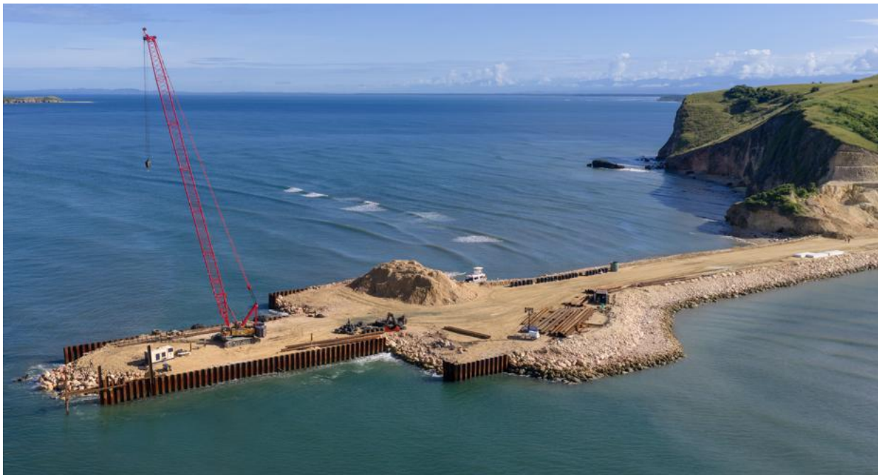
Stage 3 Construction of the Kido Wharf underway.
