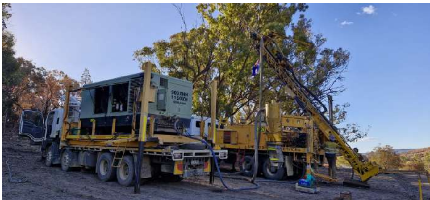
Figure 1: Drilling underway at Webbs.
