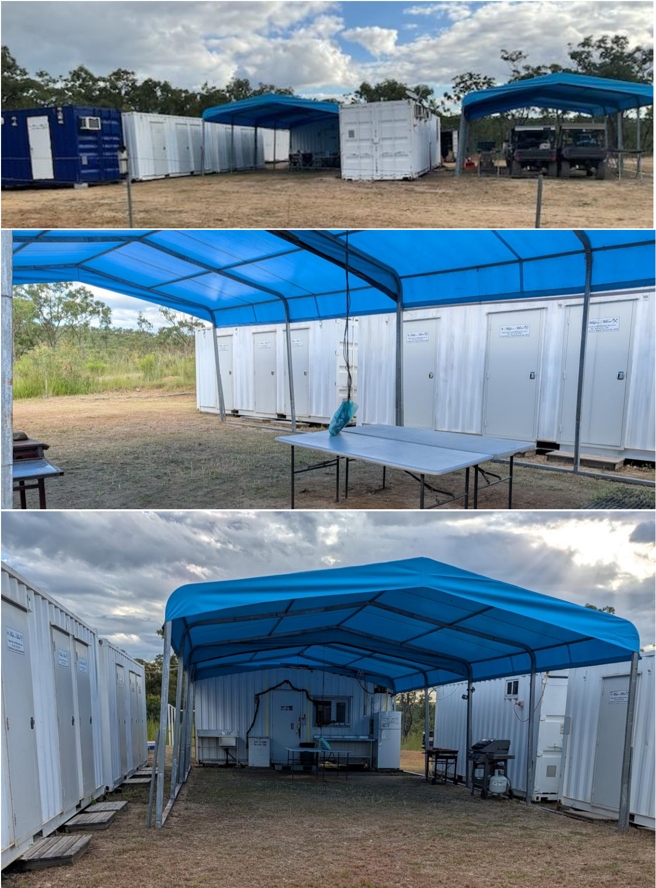
Figure 2: Upgraded and expanded Dianne accommodation village
