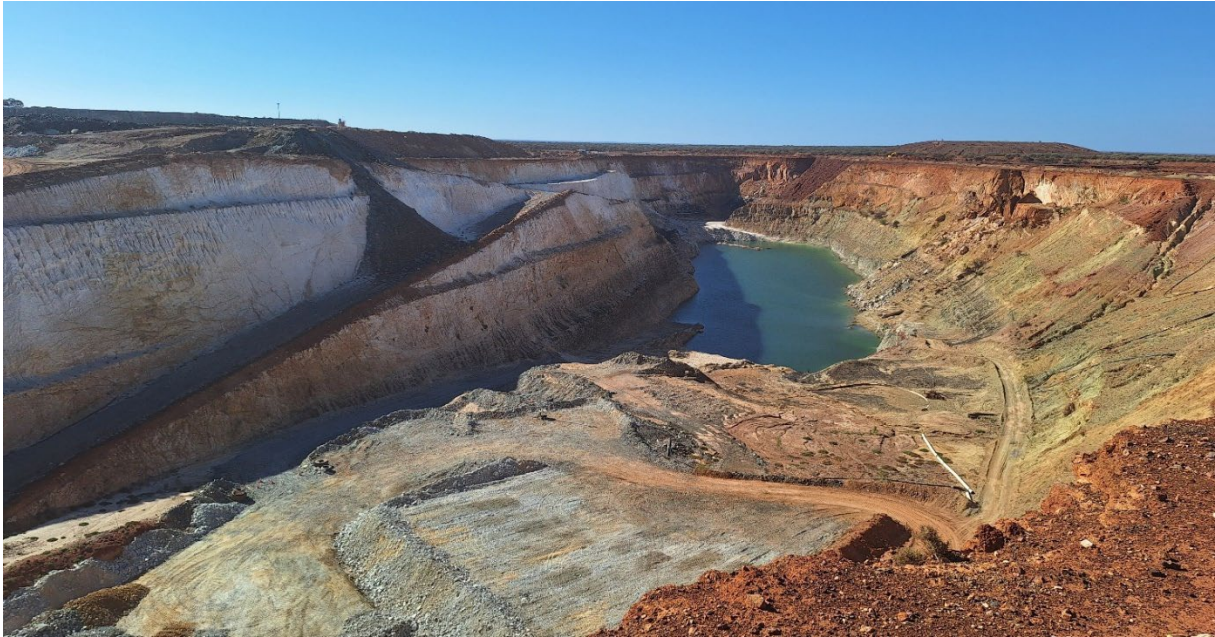
Figure 3 – Youanmi Main pit dewatering looking South (23 February 2026)
