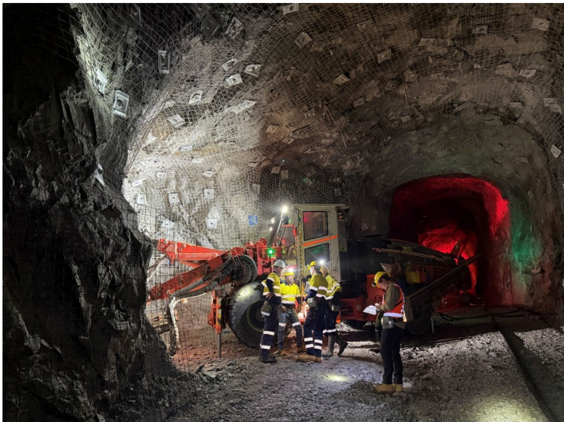
Figure 2 – Underground at United North
