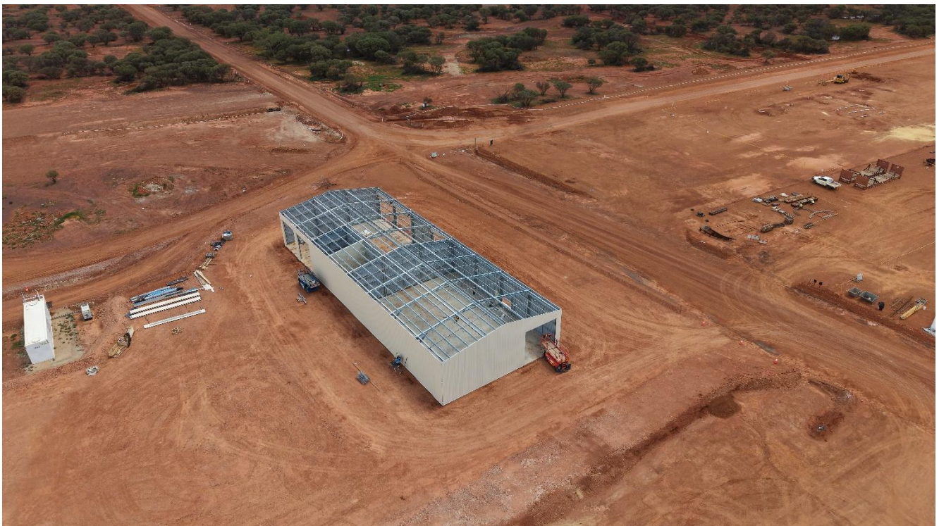
Figure 8 – Warehouse construction ongoing
