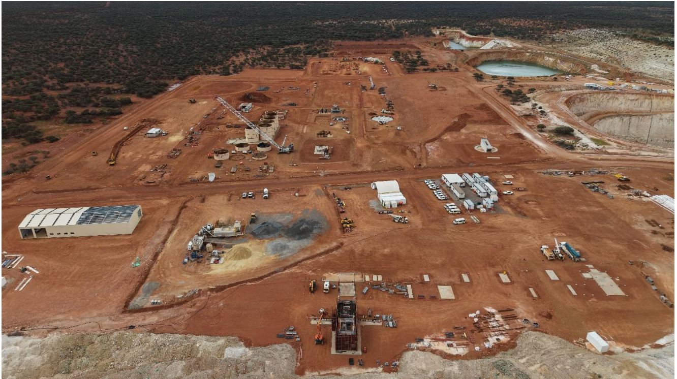
Figure 1 – Progress of construction on site – looking North
