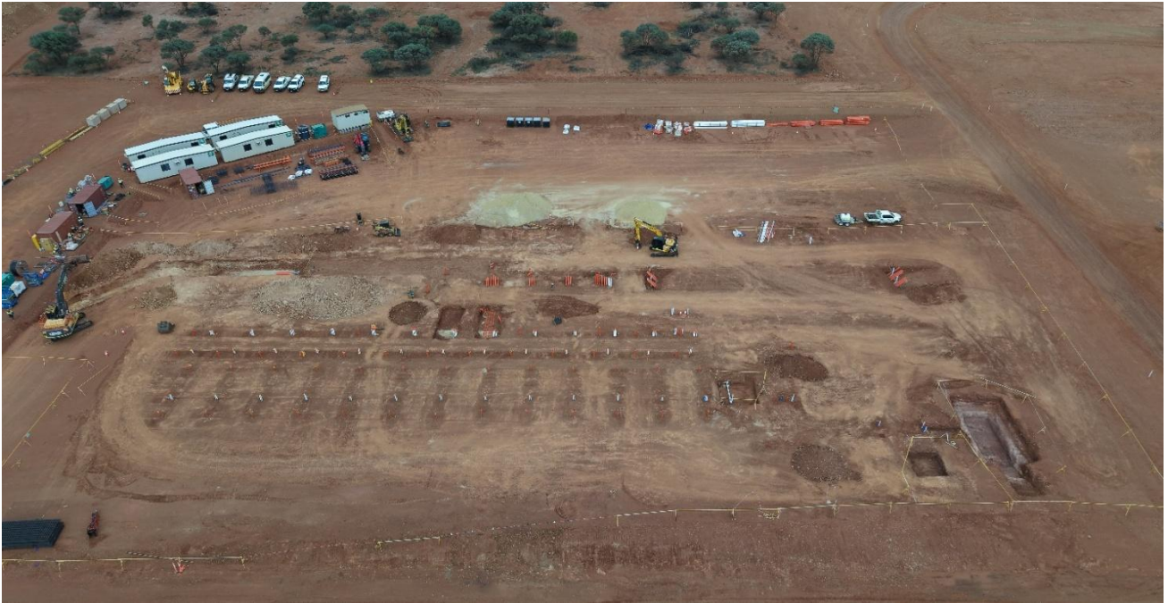
Figure 13 – Power station buried earth works
