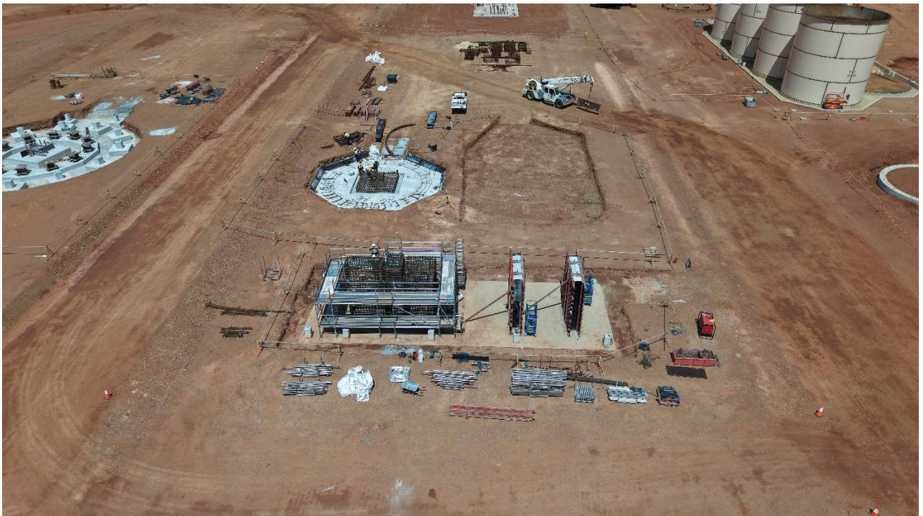
Figure 4 – IsaMill construction ongoing
