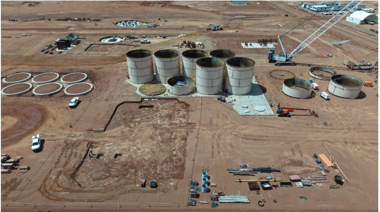
Figure 5 – CIL pad completed, tank construction advancing
