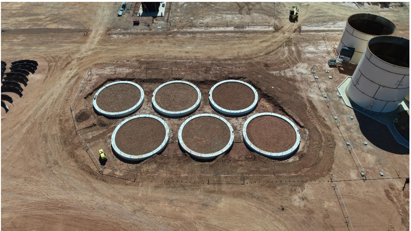
Figure 2 – Albion Tanks floors prepared
