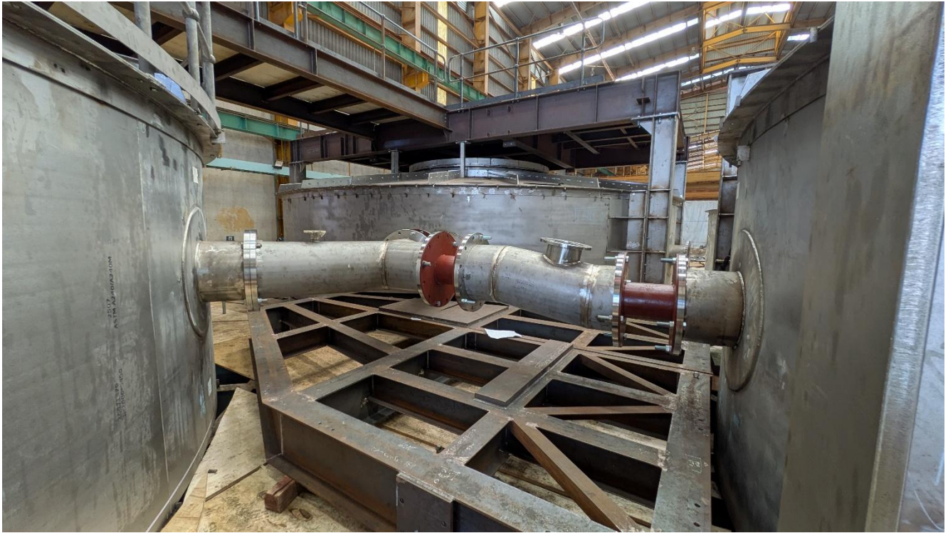
Figure 9 – Albion tanks fabrication & launder trial set up
