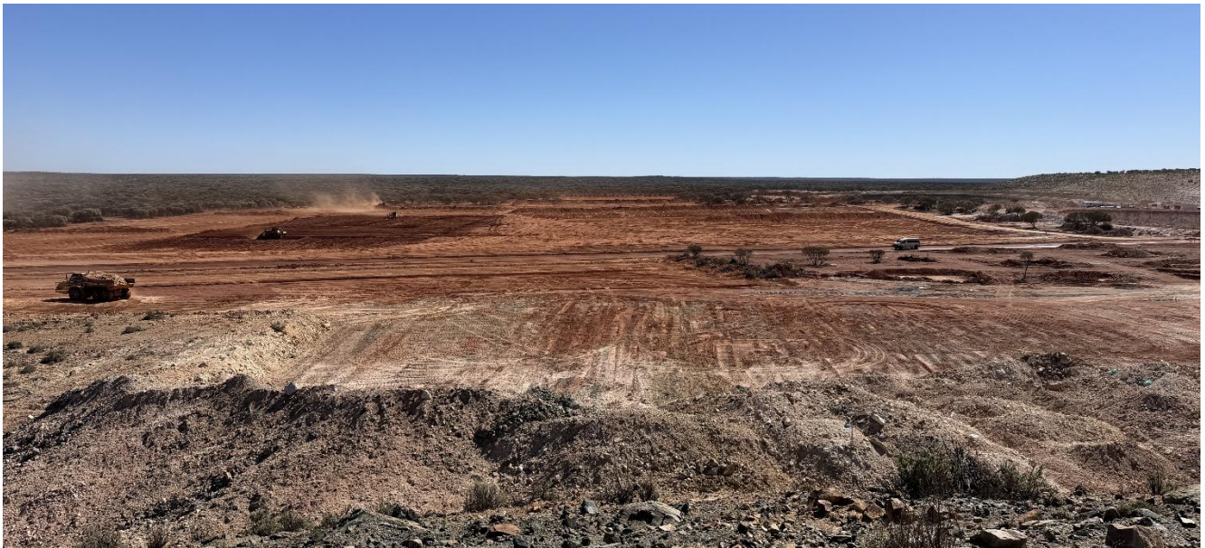
Figure 9 – Processing plant bulk earthworks underway, topsoil cleared, 1 st pad under construction
