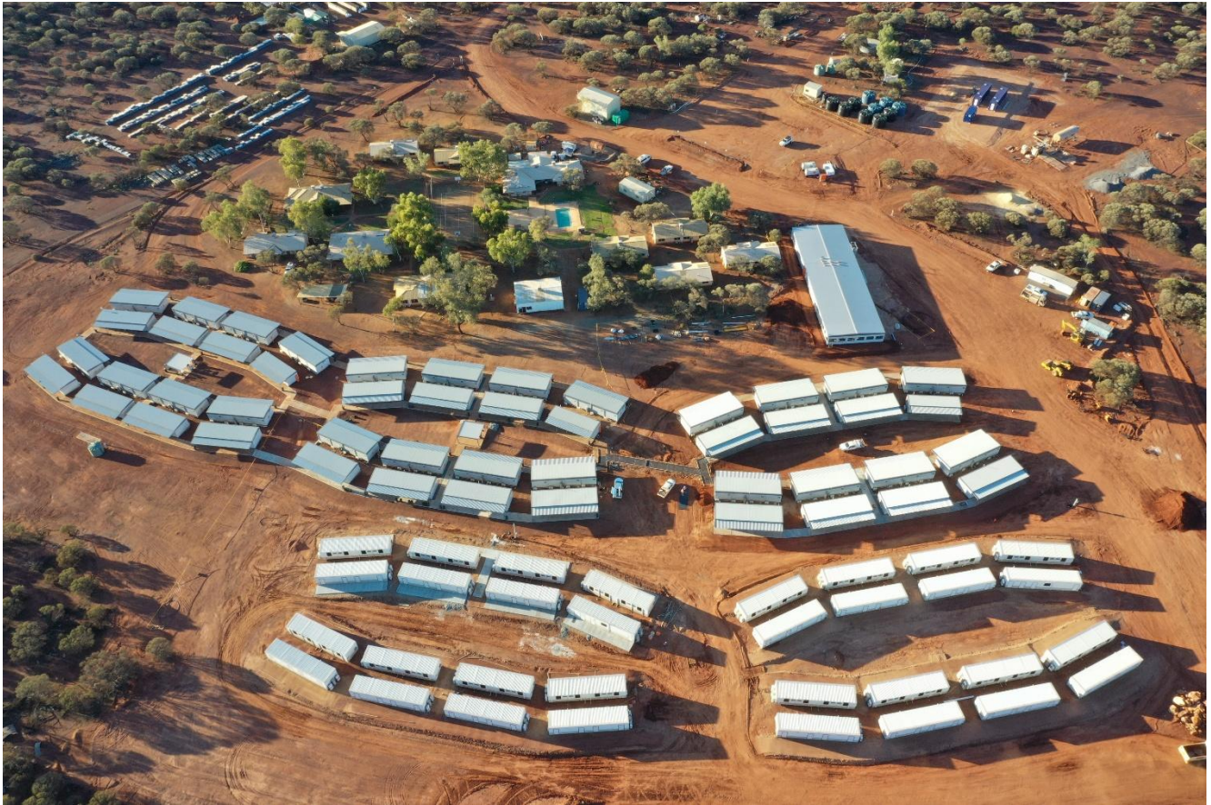
Figure 10 – Camp expansion – all buildings onsite
