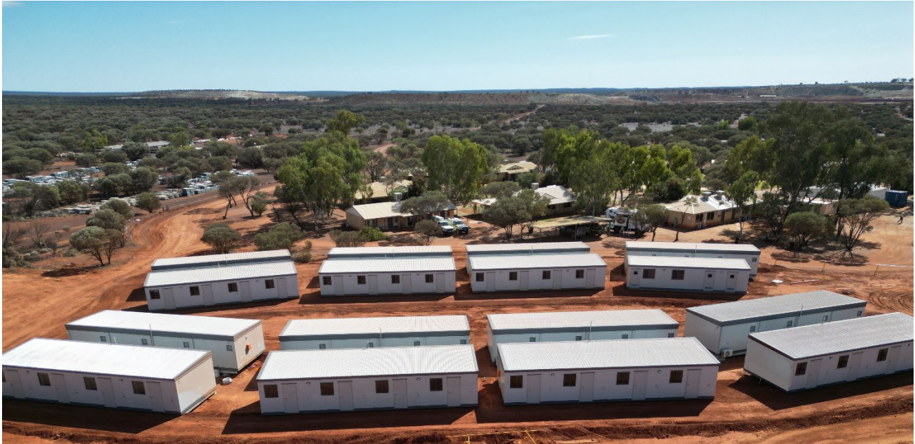
Figure 4 – Phase 1 Camp Expansion works advancing
