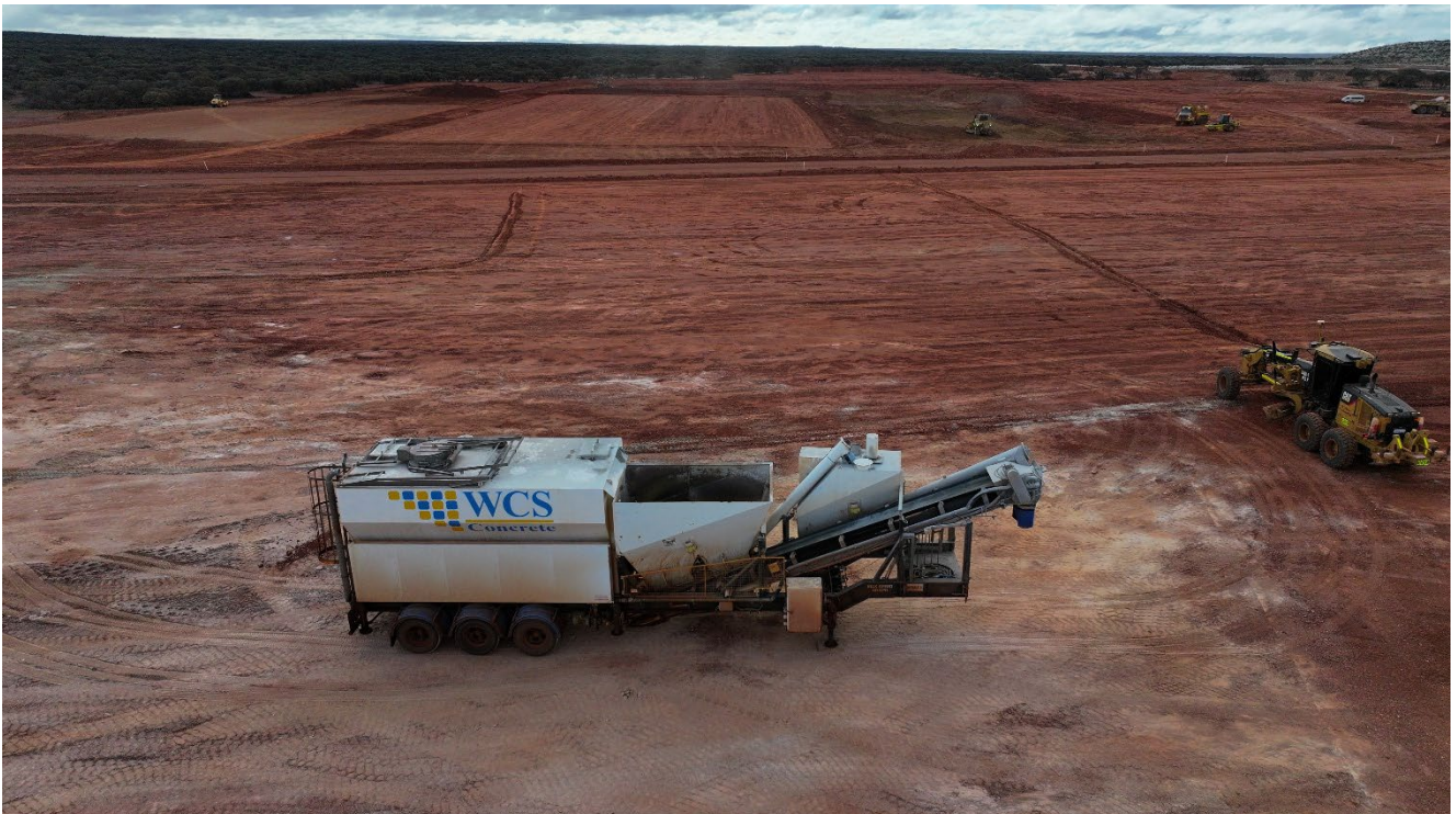
Figure 7 – Interquip Mobilisation underway
