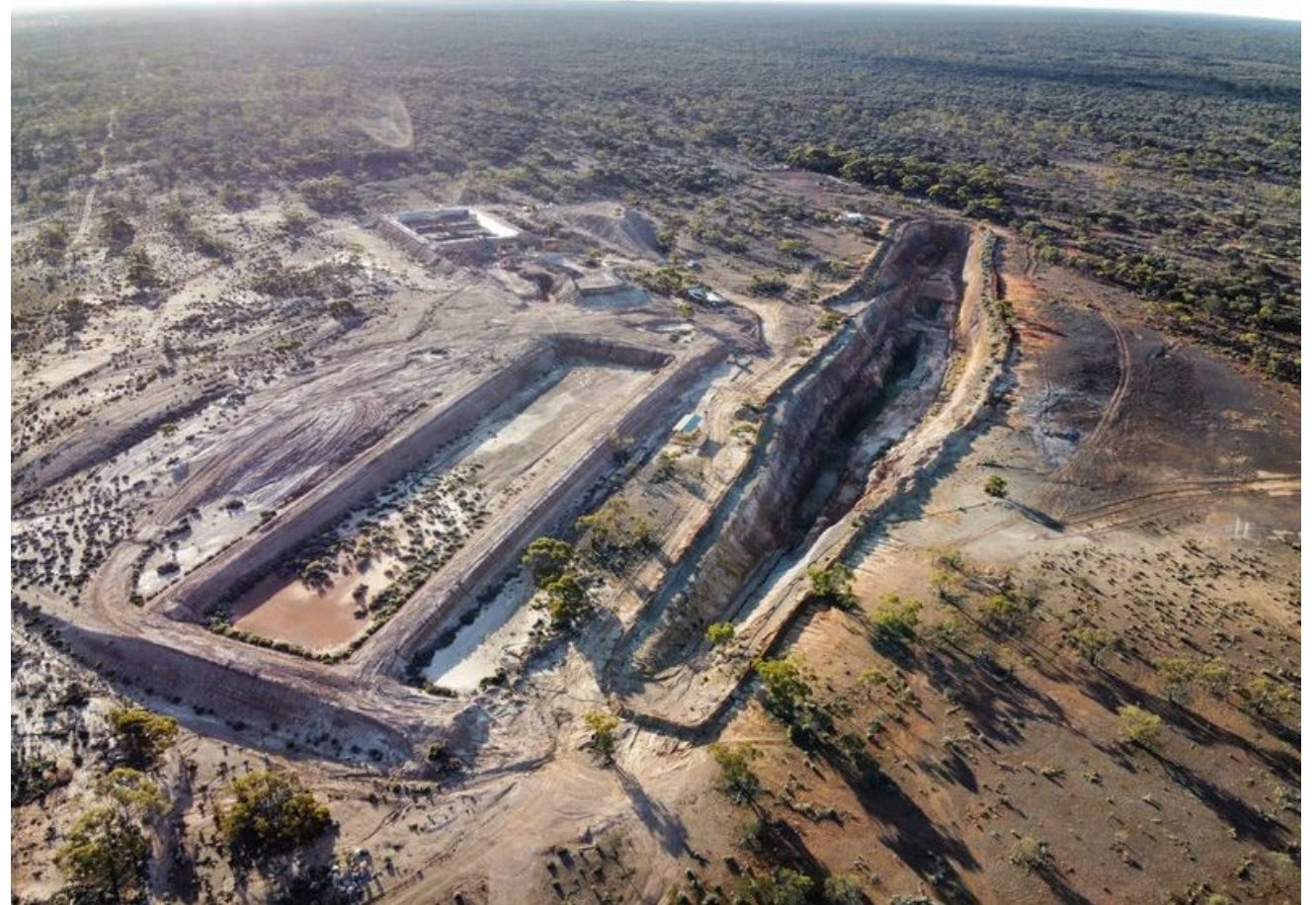
Drone photo of Zelica Project looking NNW showing pre-stripped open pit (approx. 300m long and 10-25m deep) and pre-constructed vat leach ponds (pic taken August 2025)
