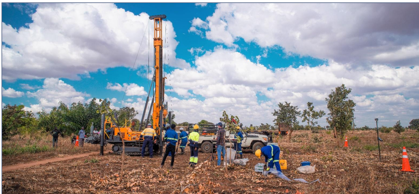
Figure 4: Core drilling (push tube) in action at Kasiya
