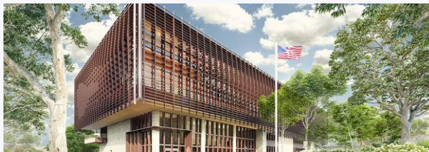
New U.S. Embassy, Lilongwe - under construction
