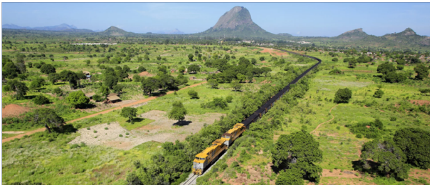
Figure 26: Bulk cargo trains operating on the NLC
