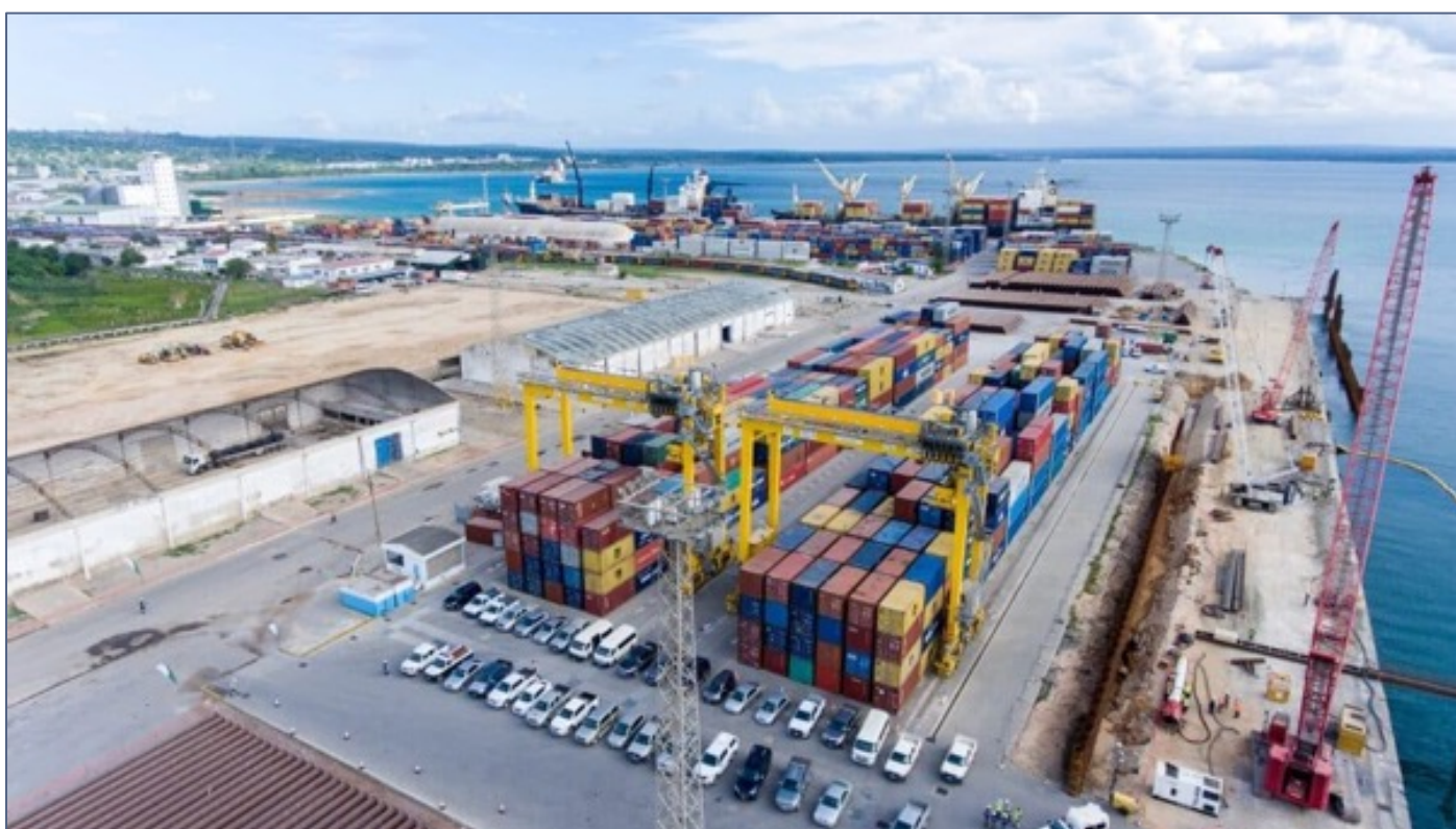
Figure 27: Port of Nacala, Mozambique
