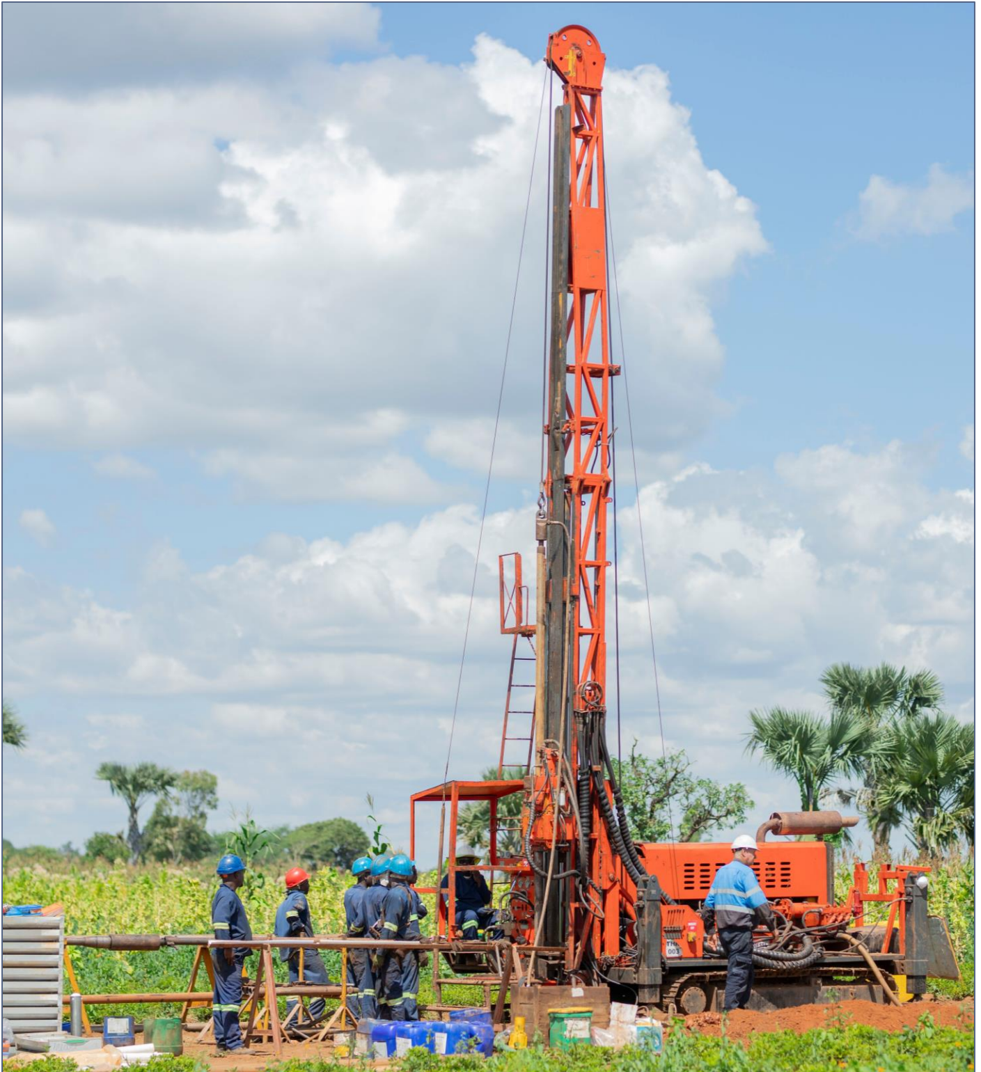
Figure 2: Geotechnical diamond drilling program underway
