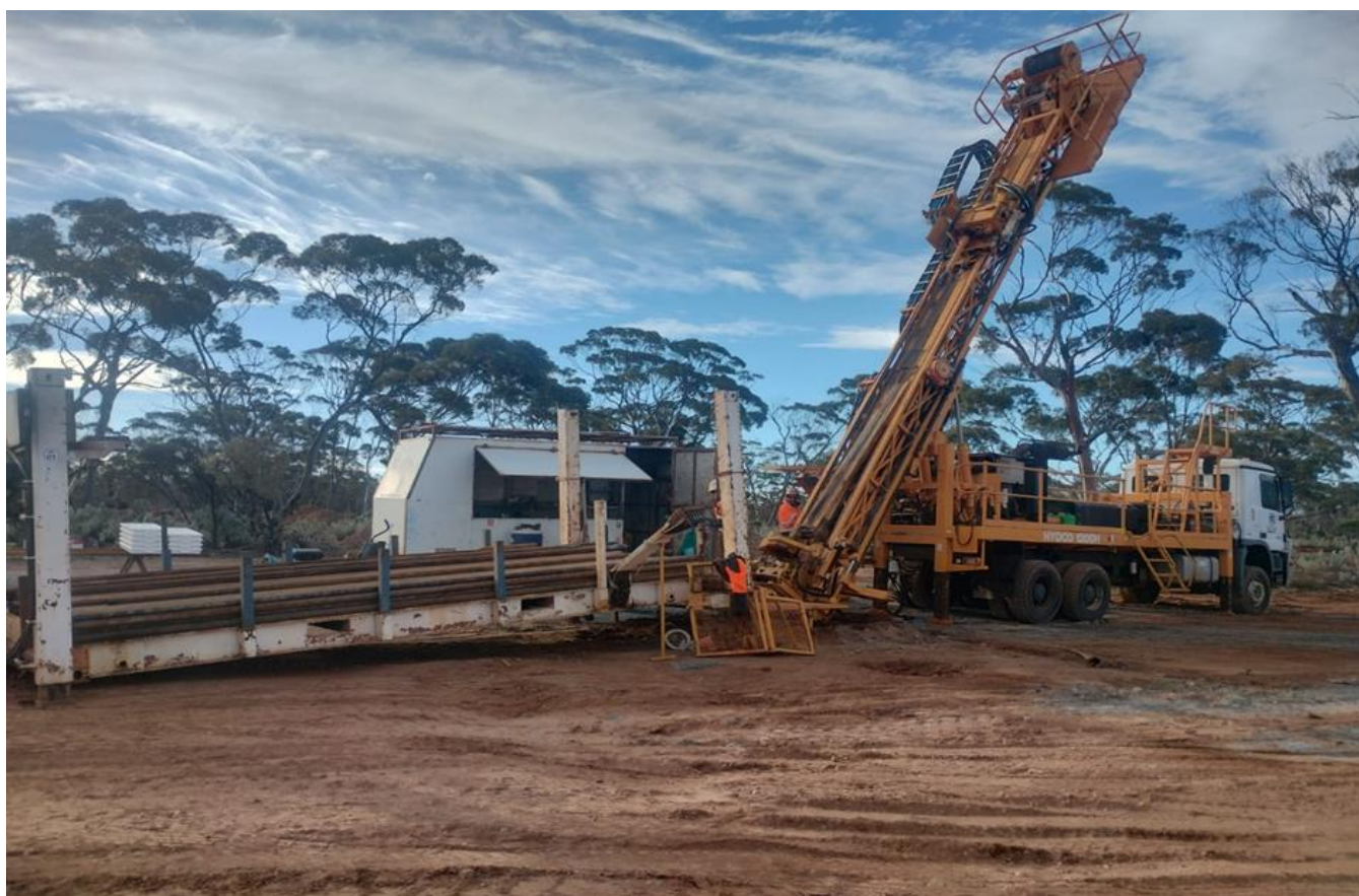
Figure 2 Diamond drilling is underway in hole 25PRC206 at the Paris Gold Project.
