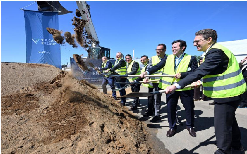
Groundbreaking at lithium chemical site in Frankfurt
