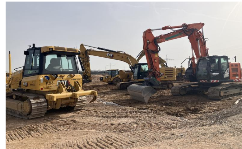
Construction at the integrated geothermal and lithium extraction site near Landau
