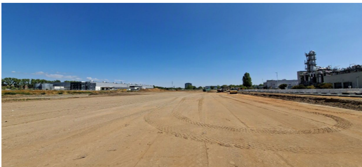
Figure 13: Early bulk earthworks in preparation for future civil activities at the Lionheart lithium chemical facility.
