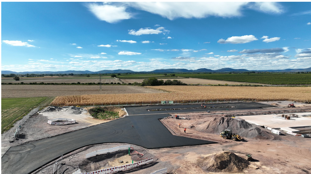
Figure 6: Aerial view of the fourth well-site under construction.
