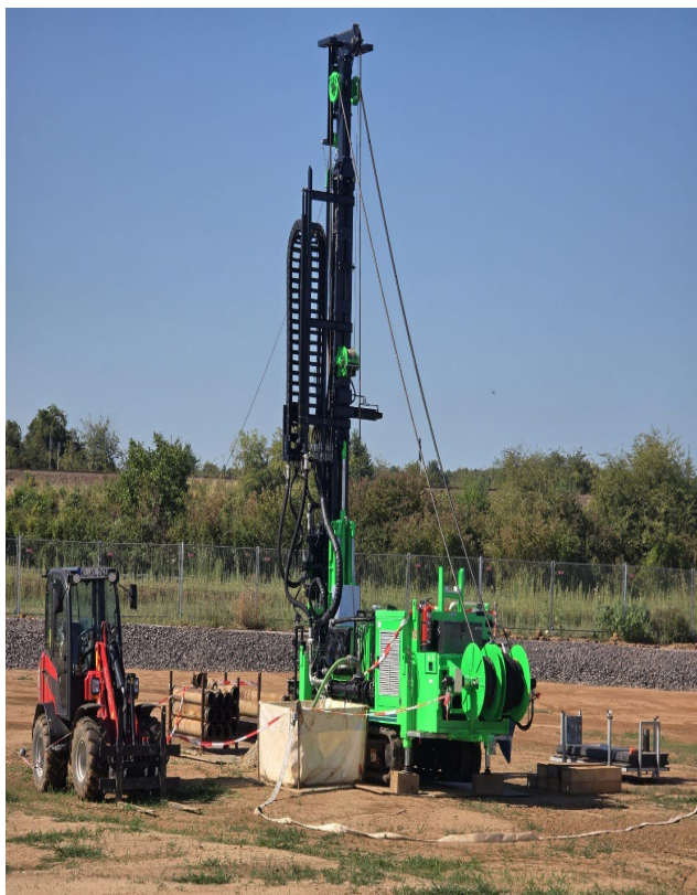
Figures 10 and 11: (left hand side) Soil investigation drilling ahead of the construction of tank foundations (right hand side) 110kV overhead transmission line which has been removed with power relocated underground.
