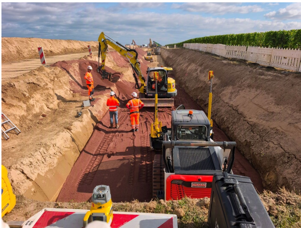
Figure 9: Trenches for Lionheart pipelines and cables to enable transportation of lithium brine and industrial water from the well sites to the geothermal and lithium extraction plant and back to the well sites for re-injection.
