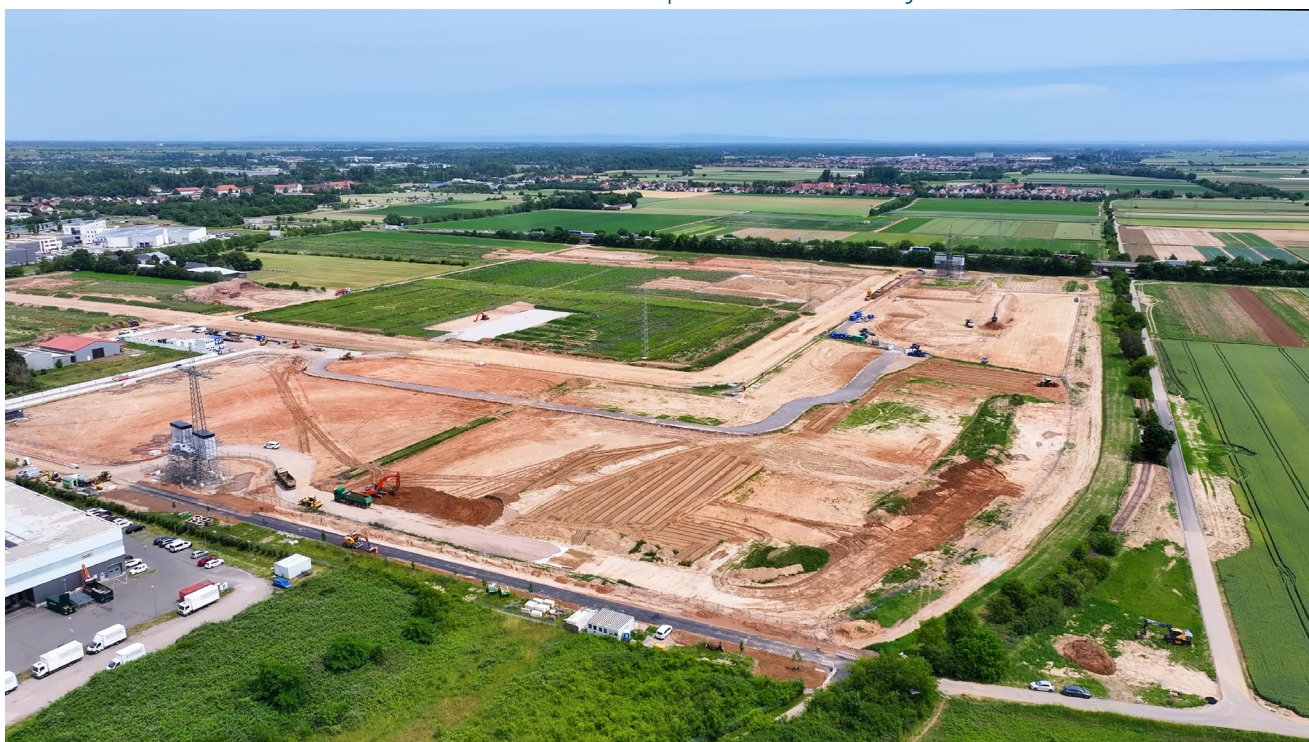
Figure 12: Site preparations at the geothermal and lithium extraction plant in Landau. See overhead powerline infrastructure which has been removed since the date of this photograph
