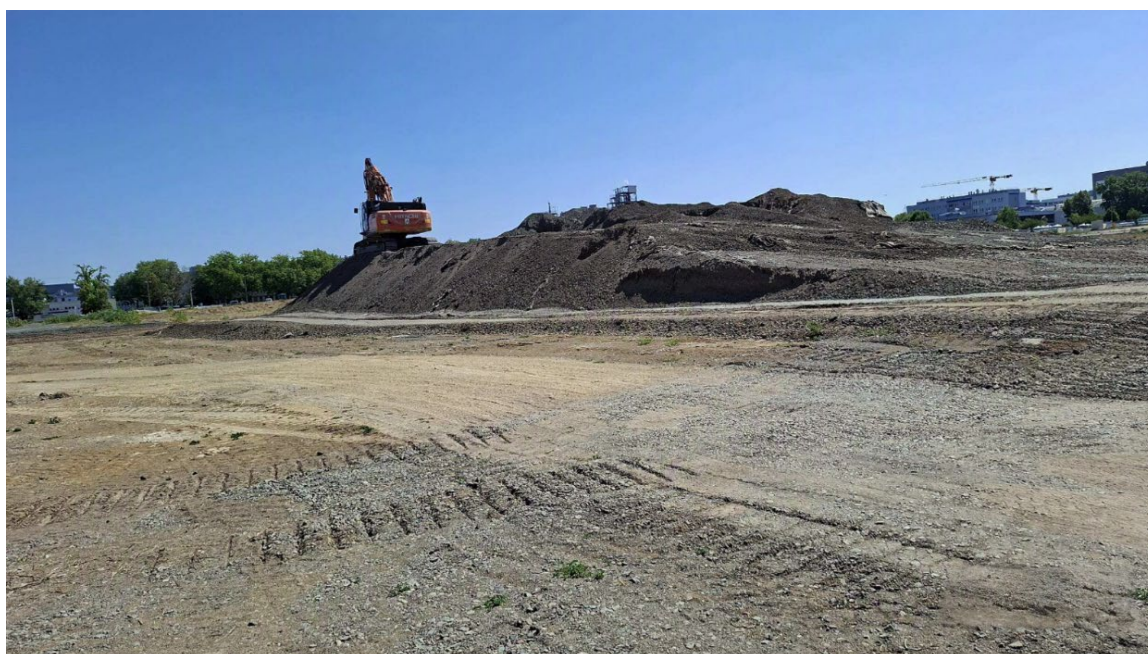
Figure 14: Early bulk earthworks in preparation for future civil activities at the Lionheart lithium chemical facility.
