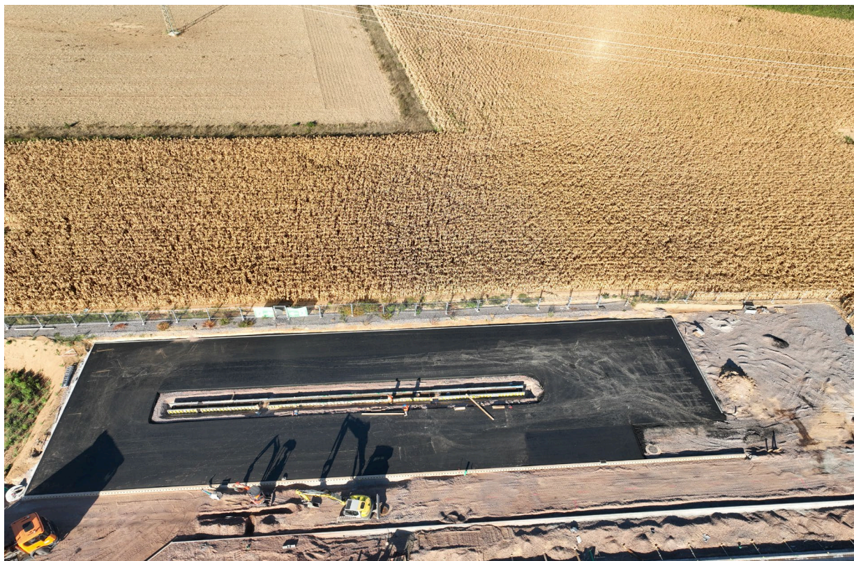
Figure 5: Construction works at the fourth well-site ahead of mobilisation of the second Vercana rig, known as V10, in Q4 2026.
