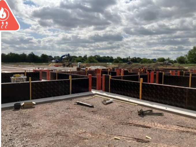
First foundation concrete layers for the Lionheart geothermal power plant in Landau
