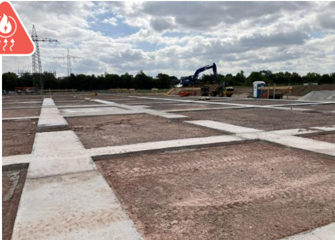
First foundation concrete layers for the Lionheart geothermal power plant in Landau
