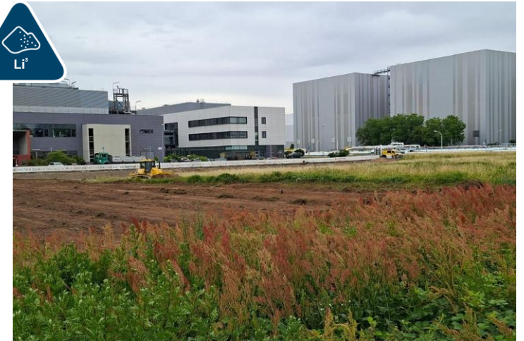
Early bulk earthworks at the Frankfurt lithium chemical plant site
