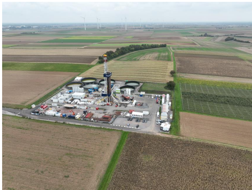
Figure 1: Schleidberg well site near Landau, Germany.
