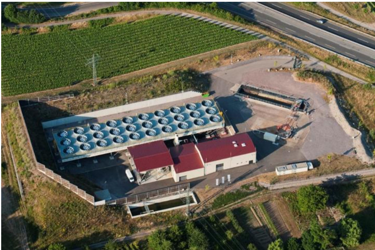
Figure 1: Aerial view of Insheim operational geothermal plant
