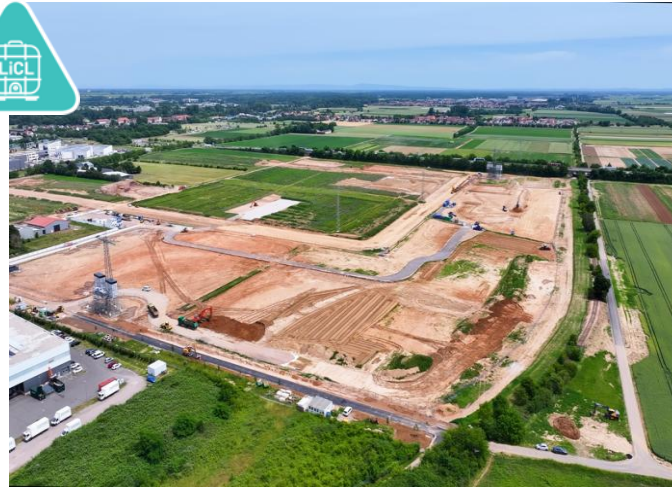
Site preparations at the Landau geothermal and lithium extraction facility. Powerlines now relocated
