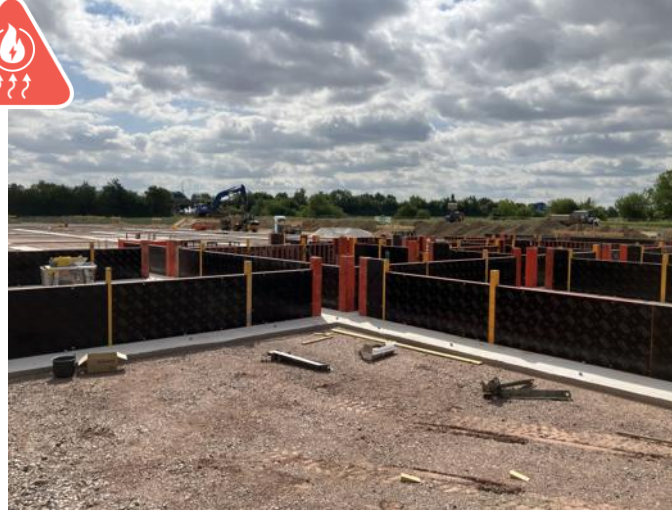
First foundation concrete layers for the Lionheart geothermal power plant in Landau
