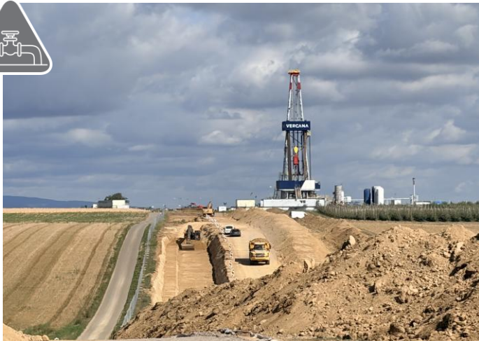
Convergence of below ground activities with construction of the above ground infrastructure supporting it
