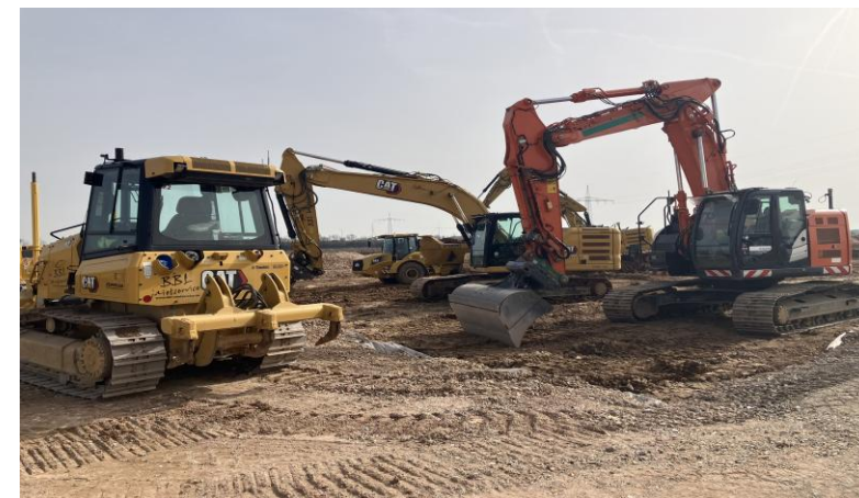
Construction at the integrated geothermal and lithium extraction site near Landau
