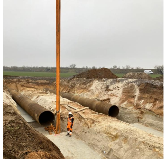
Figure 5 & 6: Concrete slabs as foundations for the duct pipes and start of installing the duct pipes (1.4m diameter) ICPP in December 2025
