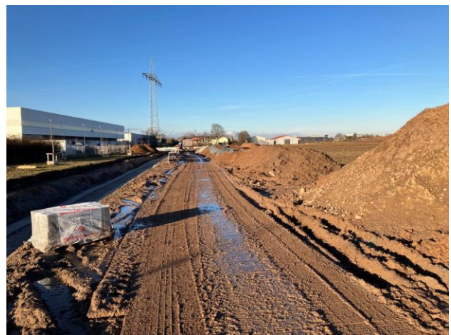
Figure 4: Preparatory works to install HV cable
