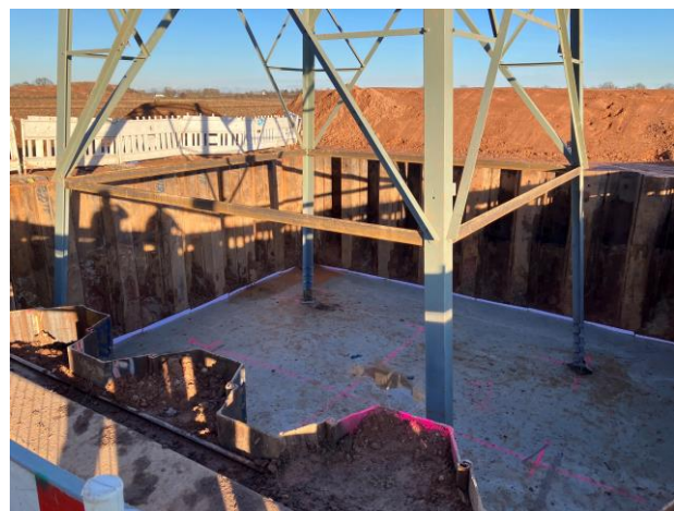
Figure 8: 110KV relocation and new pylon for ORC connection
