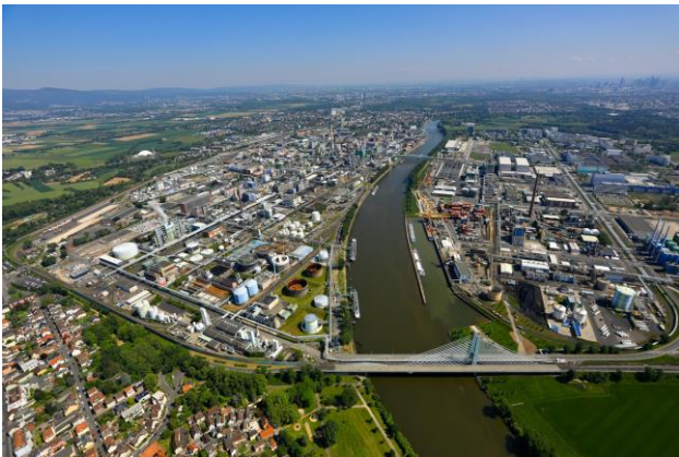
Figure 9: Infracore Park Höchst, Frankfurt
