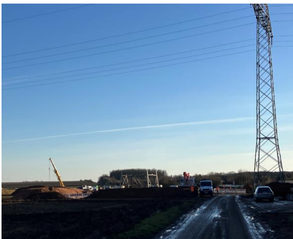
Figure 7: Earthworks at LEP site in December 2025
